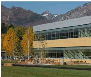
GlaxoSmithKline (photo credit: BNBuilders)
